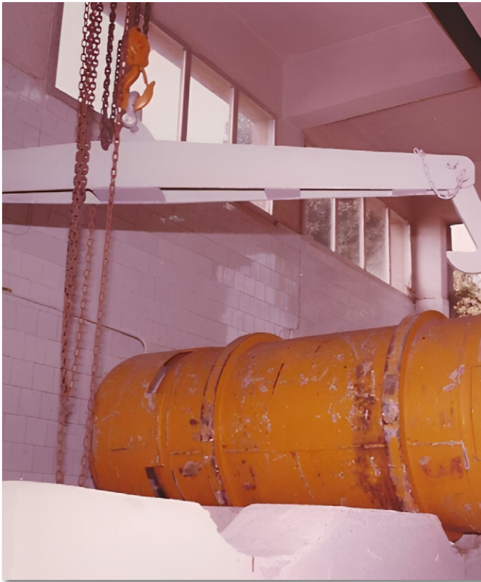
Kohafa Water Treatment Plant
