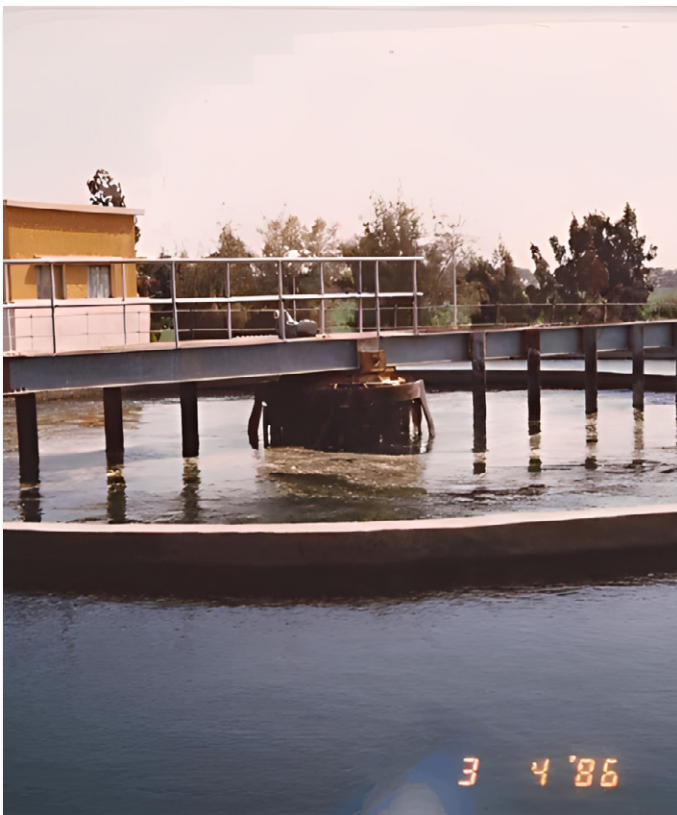
New Damietta Waste Water Treatment Plant
