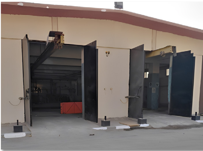
El Fostat Water Treatment Station
