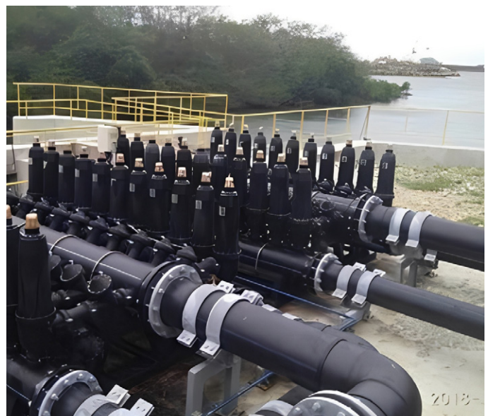
Disc-Filters System
