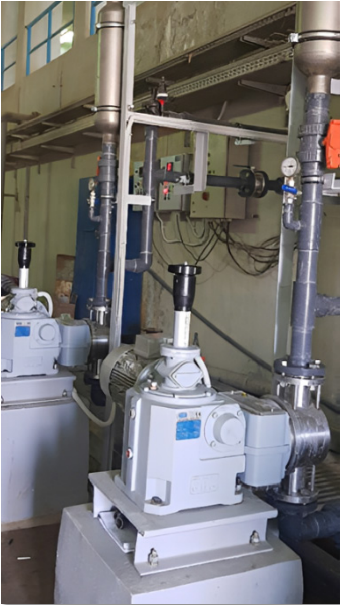
Supply & Installation of 12 metering pumps 3200 l/hr. to 4500 l/hr. for Giza WTC
