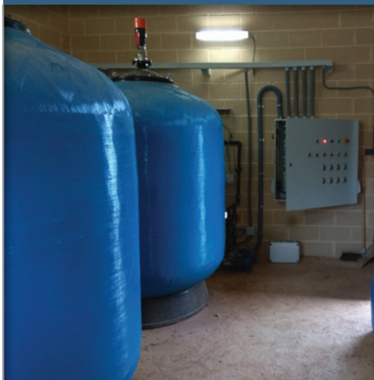
DWTP INDOOR: View of the DWTP indoor with the Bio-filers and the PLC.
