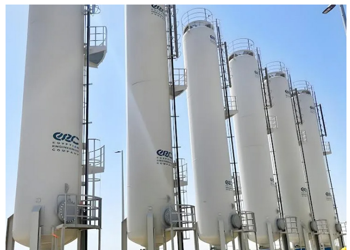
10 surge vessels with capacities 100 m 3 , 60 m 3 and 30 m 3 .
