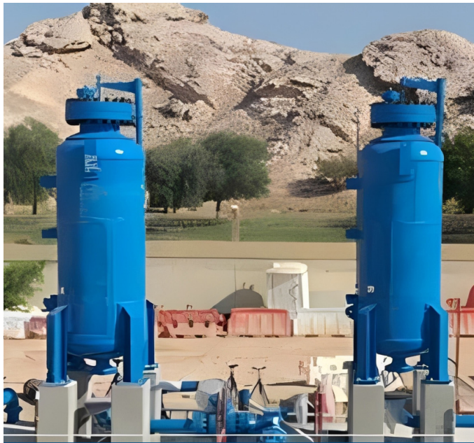
Surge vessels with design pressure 150 bar
