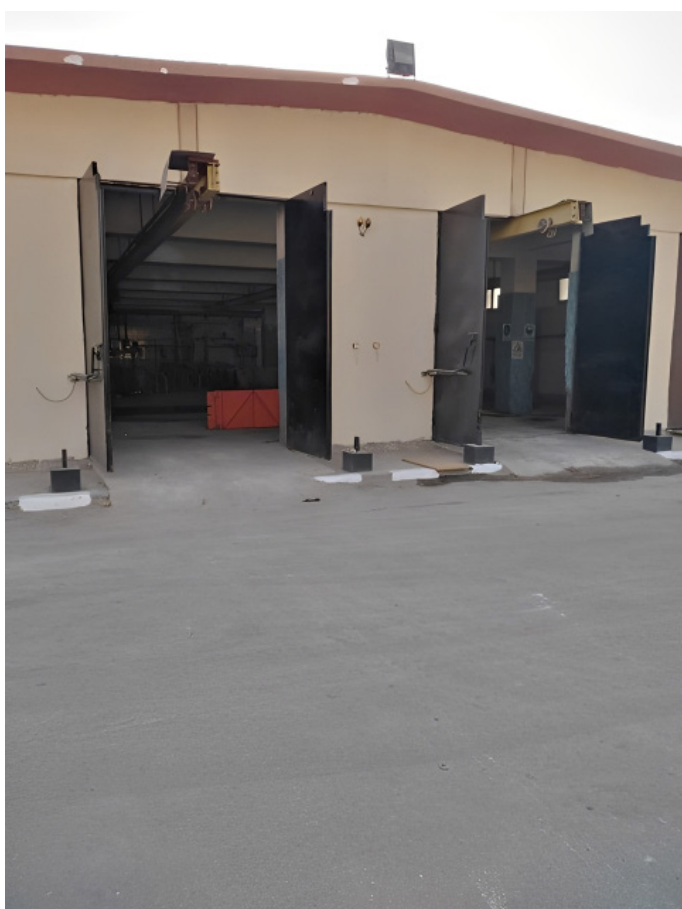
El Fostat Water Treatment Station
