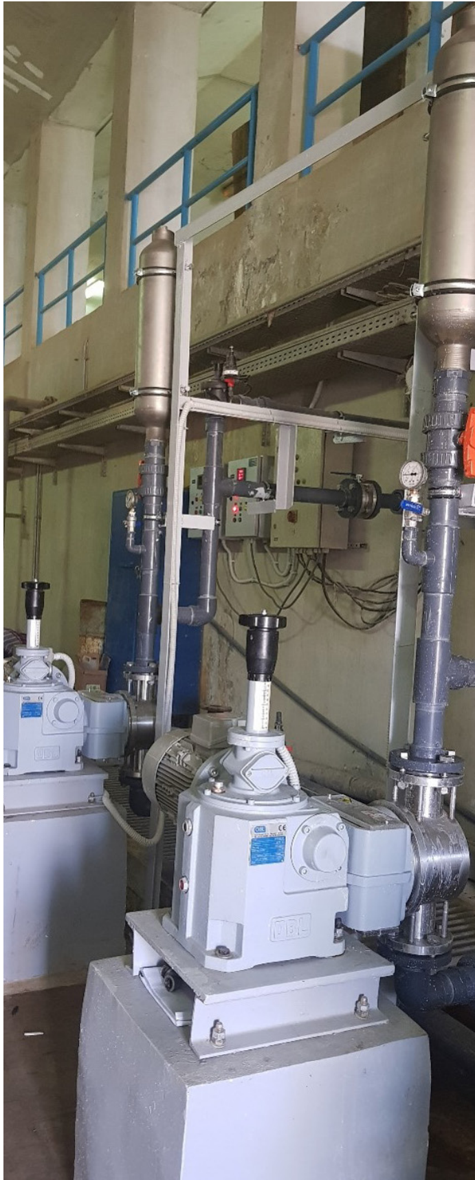
Supply & Installation of 12 metering pumps 3200 l/hr. to 4500 l/hr. for Giza WTC.
