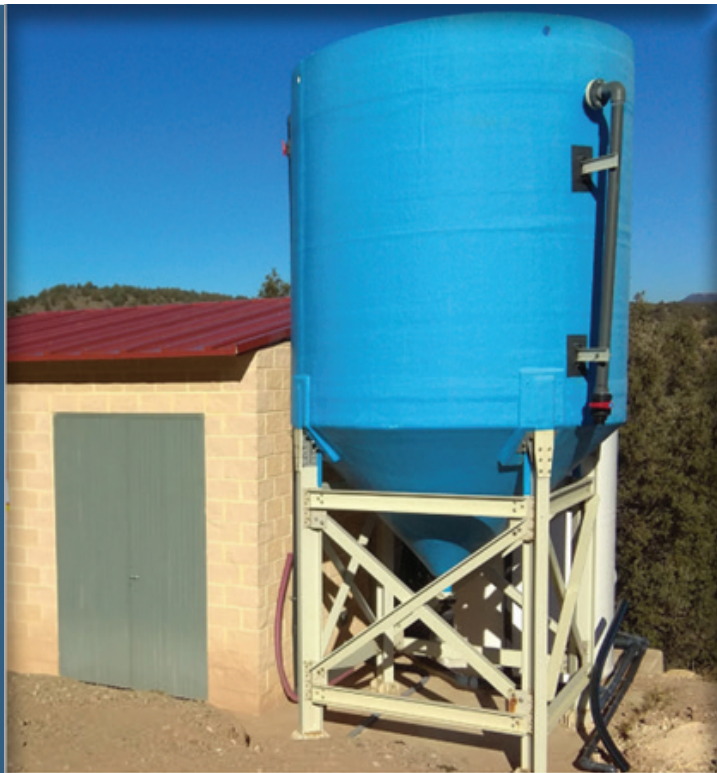
THE SMALL PLANT: View of the small plant with the sedimentation tank outside.
