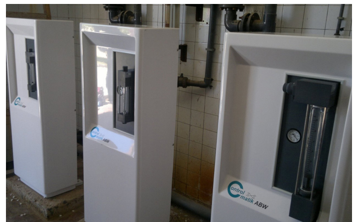
East Antara Water Treatment Station
