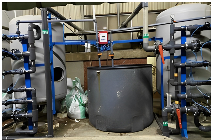
Duplex Water Softener with Multivalve System
