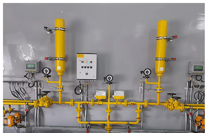
Gas Chlorination at Bahr El Bakr Project
