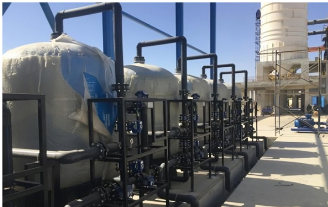
Pre-treatment Filtration System for Foreign Company
