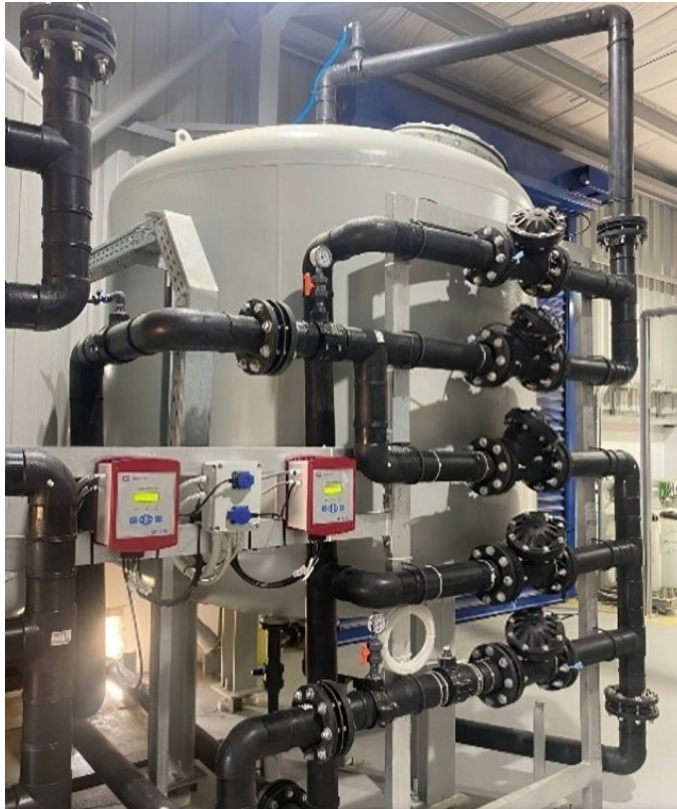
Omni-Filtration with Multivalve System
