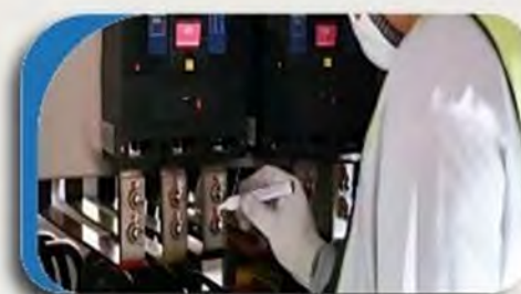
Control and Regulating Systems
