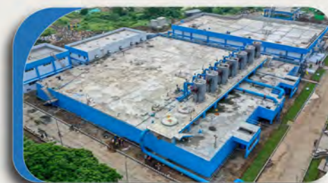
Koyambedu Water Reuse Plant
