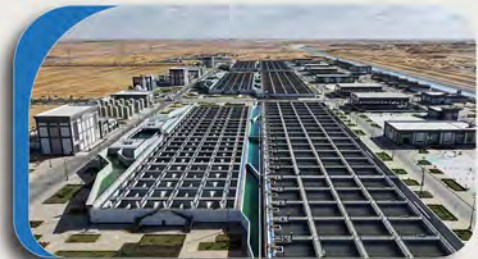
Completion of Civil and Mechanical Works And Electrical For Pumping Stations
