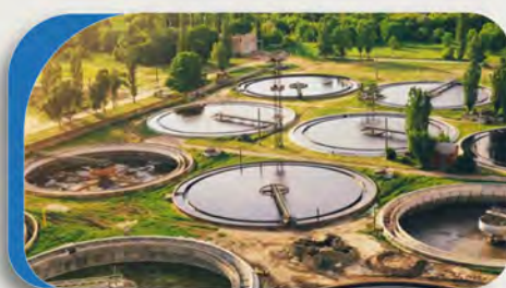
STP Sewage Treatment Plant
