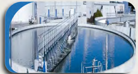
Wastewater Treatment Systems
