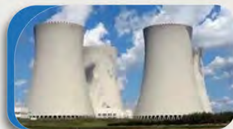
Water Cooled Chiller
