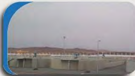
Waste Water Field
