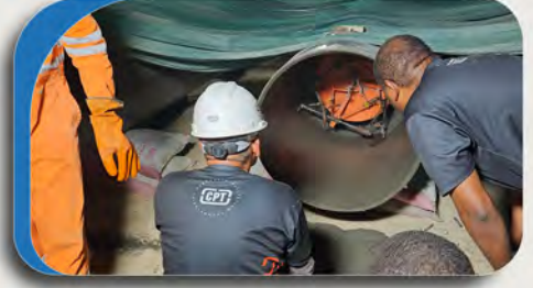
Internal Coating of Pipes
