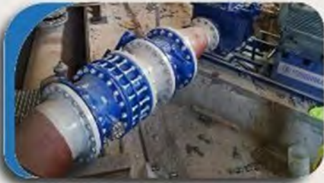
Water and Sewerage Works
