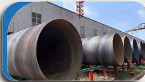
Pre-Fabrication of Piping
