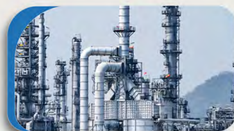
Pipelines and Pump
