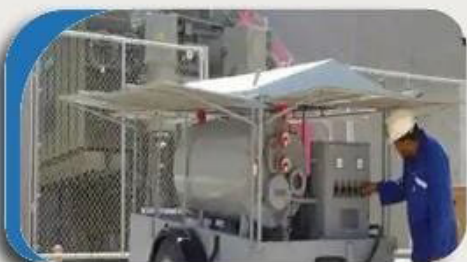
Testing & Commissioning of MV/HV Equipment
