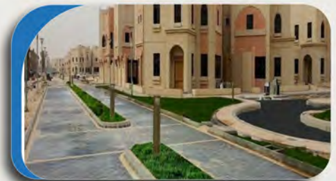
Contractors (King Faisal University)
