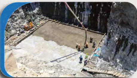
Implementation of The Sewage PipNetwork and Sewage Pumping Station With its annexes in Tayma housing project
