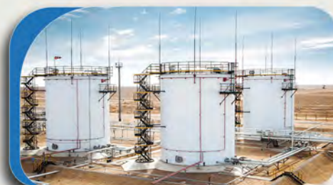
Pumping Station Construction
