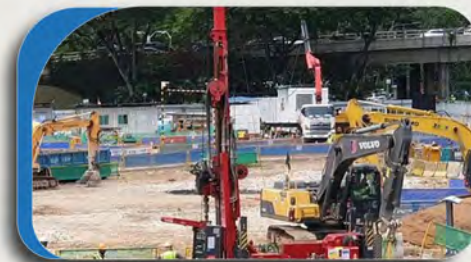
Deep Well Excavation
