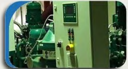
Installation of Separator Systems
