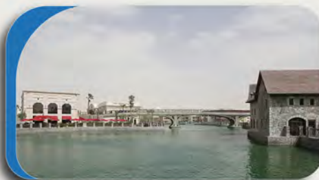
Water Treatment Systems
