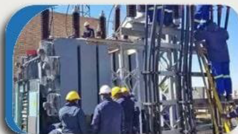
Transformer Repairing Services on Site
