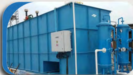
Membrane Bioreactor (MBR)
