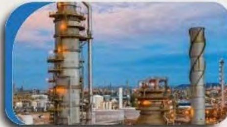
Installation of Transmitters
