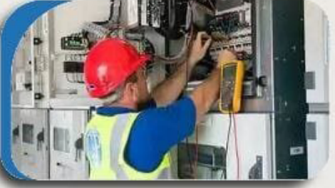
Transformer Emergency Maintenance Services
