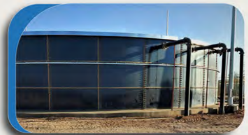
Supply and Installation of Pumps, Water Lines, and Collection Tanks for Water Conveyance From Wells Field At Salsalah & Thamad
