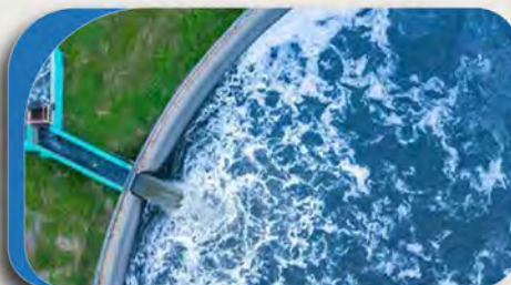
AlUla Complete Water Project
