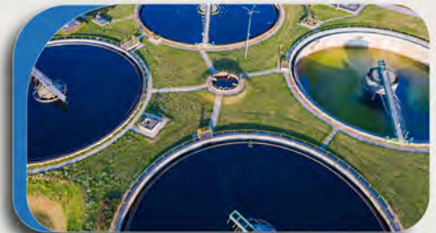
Wastewater Treatment Systems
