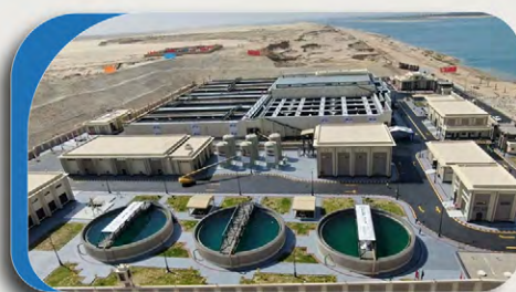
New Delta Water Treatment Plant – Egypt
