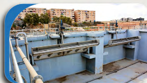
Abu Talat Sewage Treatment Plant – Egypt
