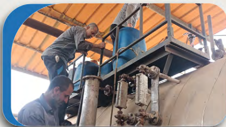
Chemical Washing Of a 10-Ton Steam Boiler
