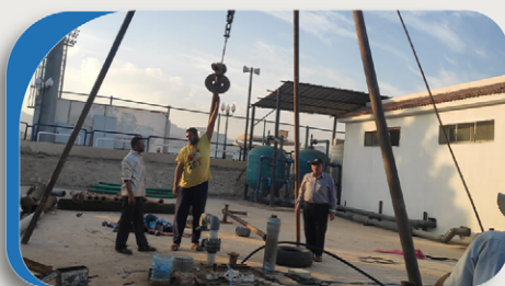
Process of Purifying and Rehabilitating Well
