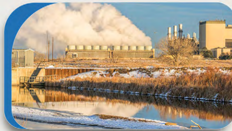
Industrial Wastewater Treatment
