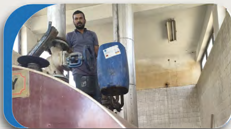
Chemical Cleaning Of The Steam Boiler
