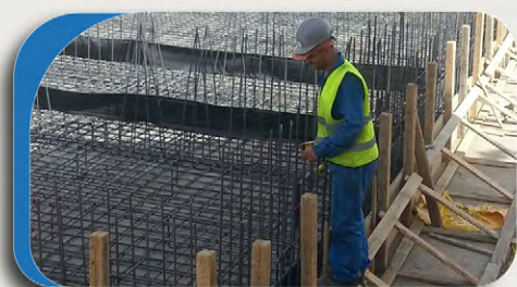
Primary Treatment Unit
