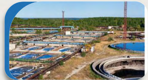
Industrial and Pharmaceutical Water Desalination Plants
