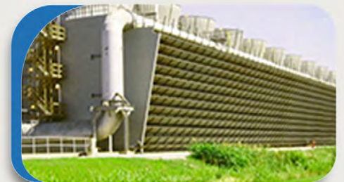
Water Cooled Chiller
