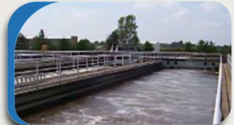
Water Treatment Systems
