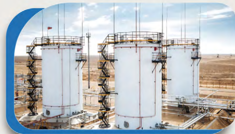
Pumping Station Construction
