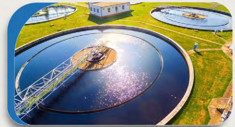
Municipal Waste Water Treatment
