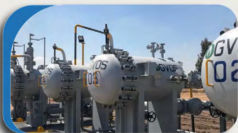
Wastewater Treatment Systems
